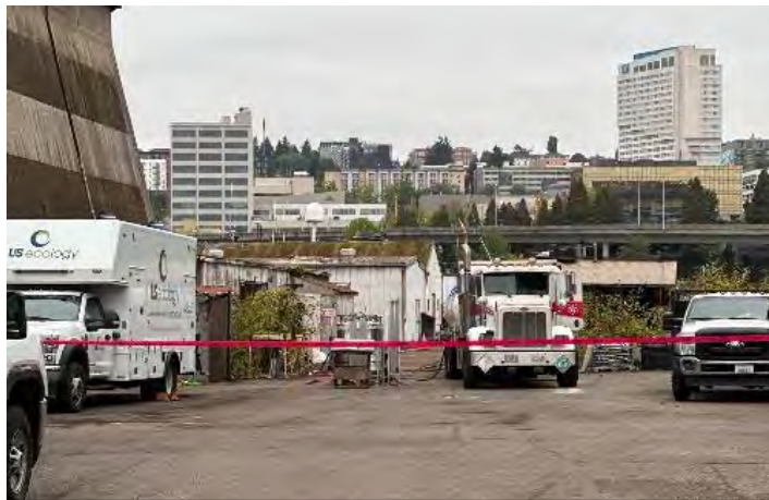
Vac Trucks removing Anhydrous Ammonia
