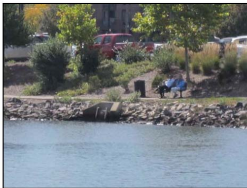
Culvert located near National Grid
